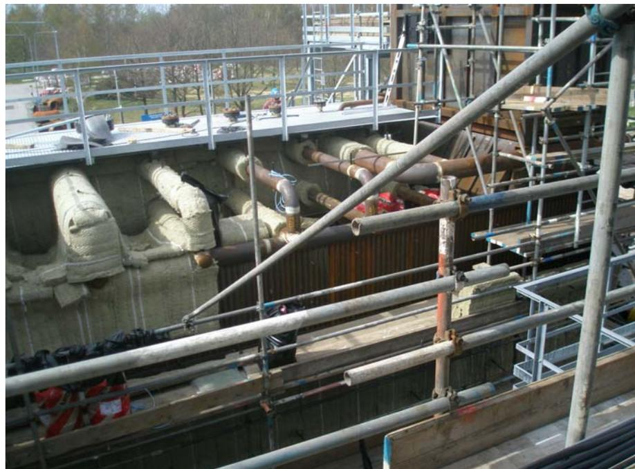
*Figure – Erection of 30 MW<sub>th</sub> boiler for saturated steam. In this case it is an outdoor installation (Stenungsund)*
