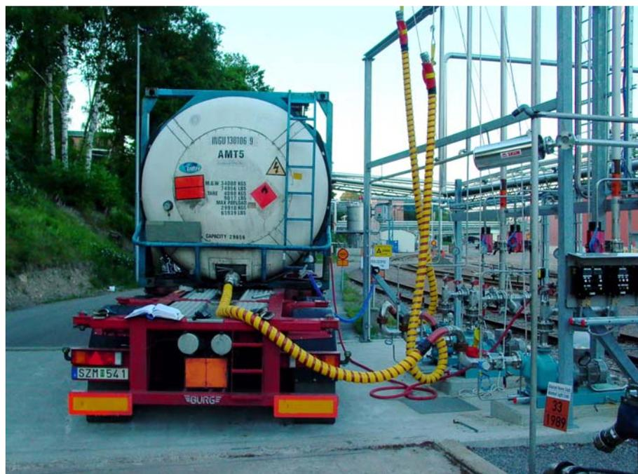
*Figure – Receiving station for hazardous waste.*
