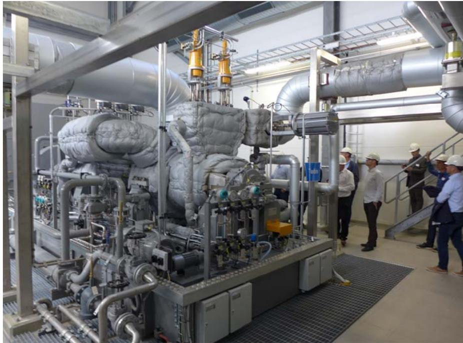
*Figure – Typical small turbogenerator installation (Nybro)*
