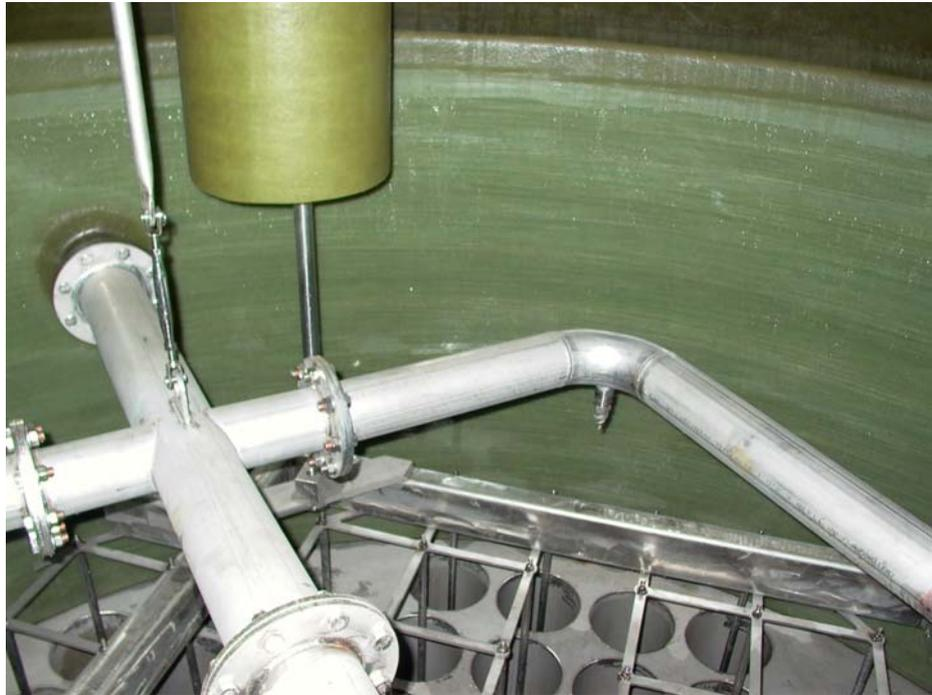
Figure – Interior from wet electrostatic precipitator.
