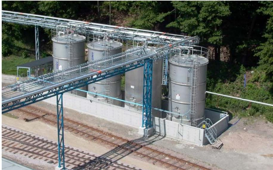
*Figure – Storage tanks for hazardous waste. Several different types can be mixed simultaneously.*
