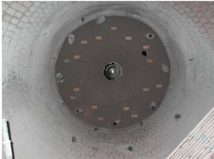
*Figure – refractory lining of adiabatic incinerator.*
