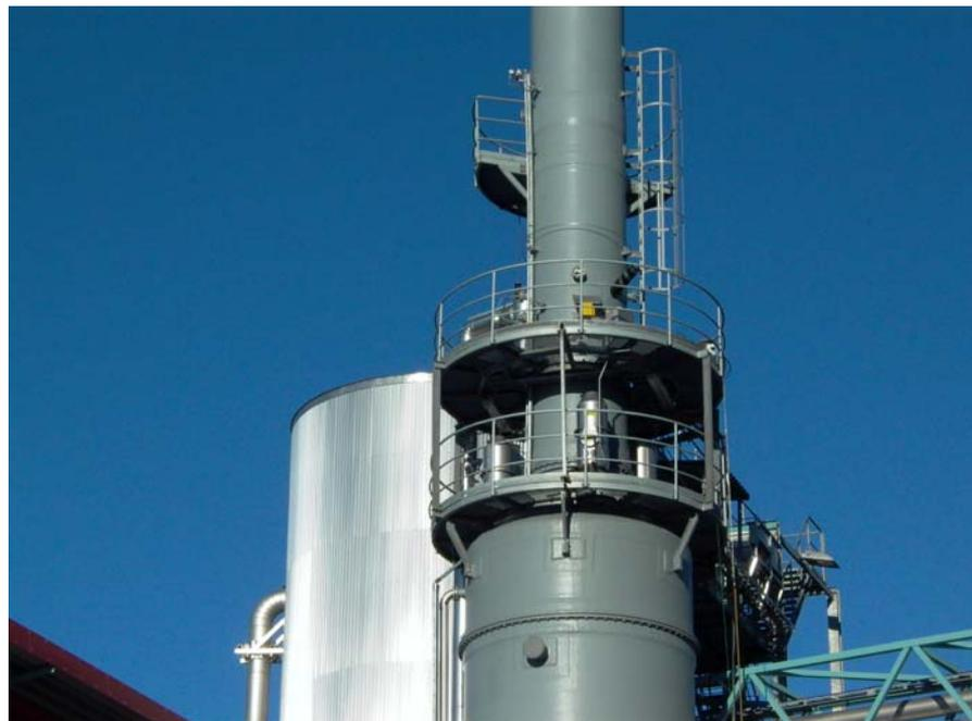
*Figure – Exterior of combine scrubber and wet electrostatic precipitator. This unit is built in GRP/ epoxy and is 65 meters high but can be built lower (Perstorp)*
