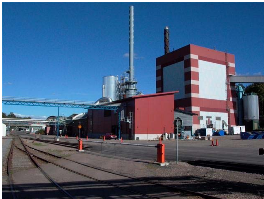
Perstorp, Sweden. Hazardous waste incinerator with WESP and animal by-products silo in the foreground. 55 MW CFBC in the background.
