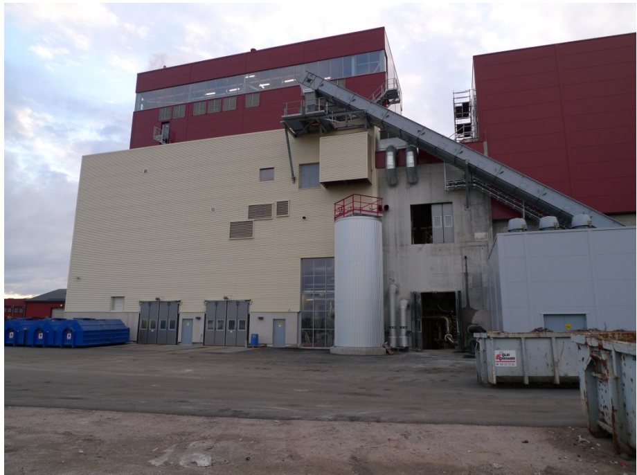
Bio-El Fredrikstad. CHP 20 MW th 6 MW el . Also possible to operate with vacuum condenser.
