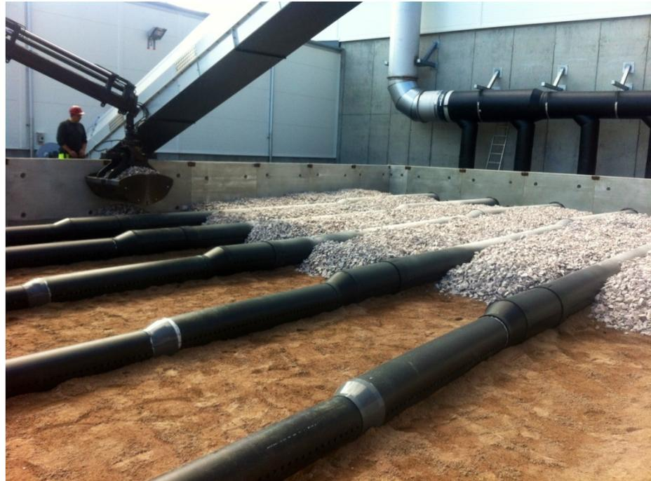
*Figure – Bio Filter for 30.000 m<sup>3</sup>/h off gases for a waste incineration plant in Västervik, Sweden during construction.*
