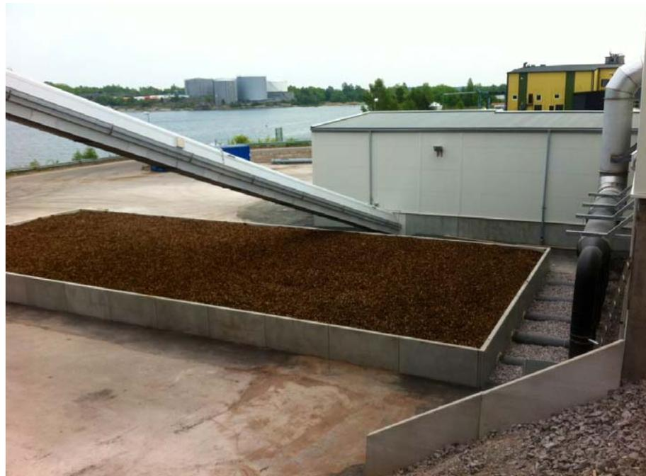
*Figure – Overview of the Västervik filter. This plant is situated by the sea some 250 meters from a residential area in the idyllic town of Västervik. Before installation of this filter, there were massive complaints of odour from an elderly installation.*
