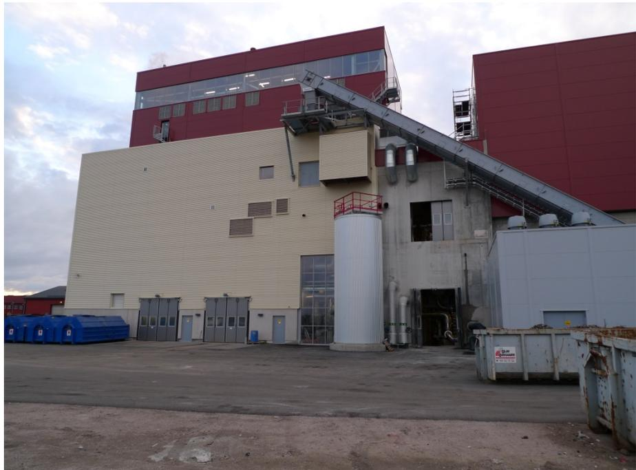
*Bio-El Fredrikstad. CHP 20 MW<sub>th</sub> 6 MW<sub>el</sub>. Also possible to operate with vacuum condenser.*
