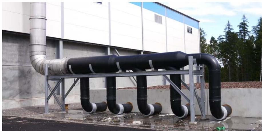
*Figure – Polluted air from fuel storage/ preparation at the waste fired plant in Nybro. The capacity is 30.000 m<sup>3</sup>/h.*
