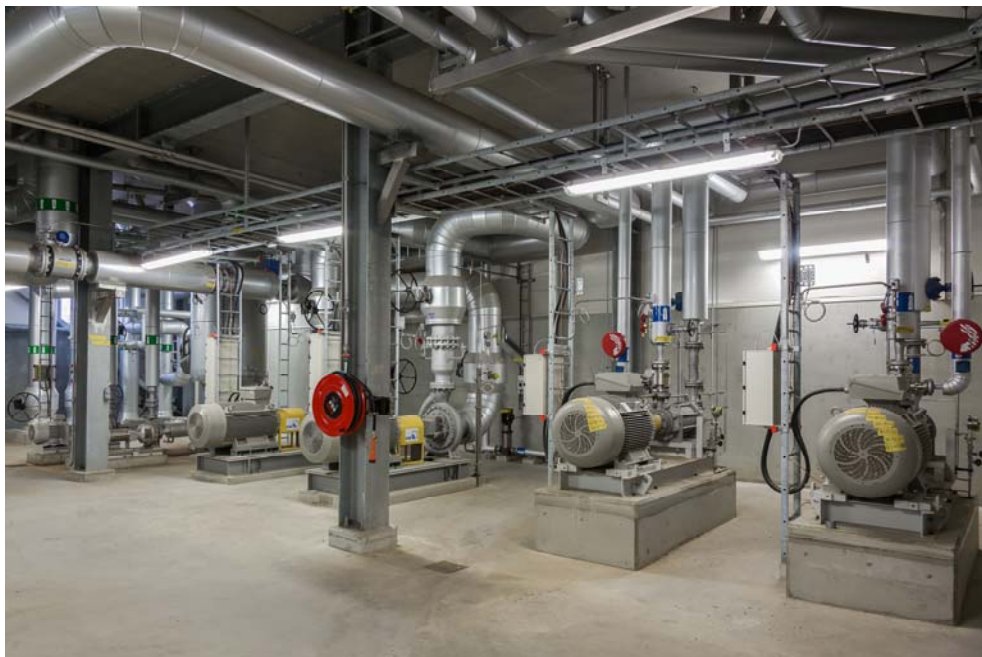
Pumpinstallation fjärrsystem – KVV Transtorp, Nybro Energi.
